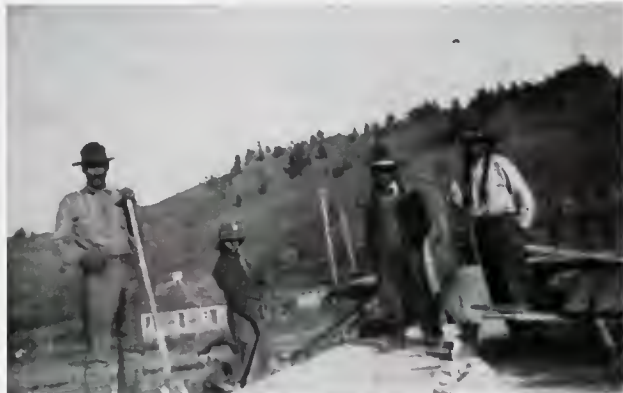
The first jail being built in 1923
